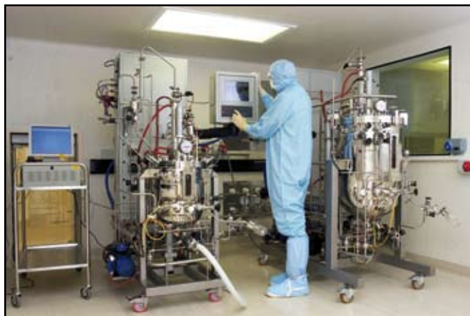
1200 x 600mm prismatic supplied to Cramlington Processing Facility, Northumberland
