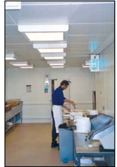
A slimline appearance is achieved by specifying a chamfered edge detail on these Surface T5 600 x 600mm luminaires with prismatic diffuser supplied to the kitchens at the Orangery, Kew Gardens.
