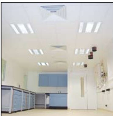
Earth Science Dept. Hoare Lea 600mm 2 T5 MRL2 louvred luminaire with (TG) toughened glass cover
