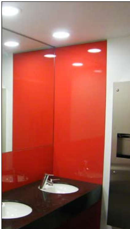
Energy efficient low maintenance lighting
